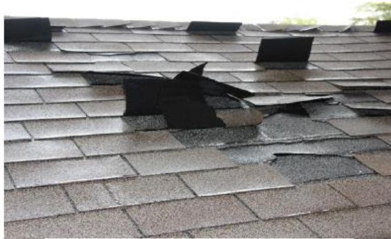
Untreated deck after 115 and 120 mph, 0 degrees. Shingles detach from adhesive strip and move back and forth with the wind until they rip.
