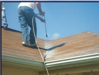
Roof-Guard being applied in March of 1999 after the cleaning
