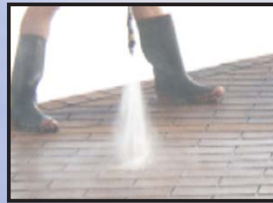
Prior to the application of Roof-Guard this roof was thoroughly cleaned.
