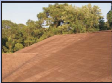
Six year old roof with mold, algae and mildew this photo was taken in Spring of 1999
