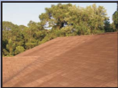
Six year old roof with algae this photo was taken in Spring of 1999
