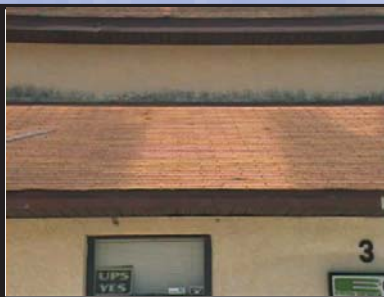
This is a test section of our Factory where Roof-Guard was applied in April 1999. This photo was taken in June of 2004
