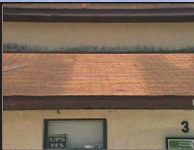
This is a test section of our Factory where Roof-Guard was applied in April 1999. This photo was taken in June of 2004
