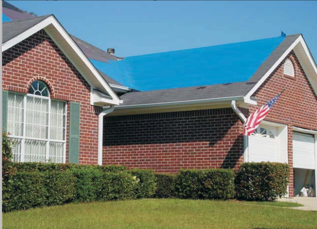
Typical of the neighbors roofs, all 24
