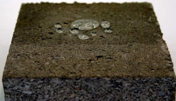
Water Test on Sealed Concrete
