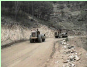
Final compacting w/25ton
