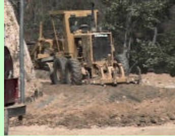
Mixing rock, sand and silt and 2001 with Cat 14w/ripper
