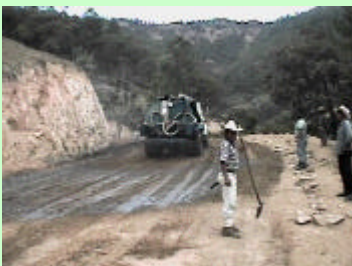
Spraying on the 2001 for mixing
