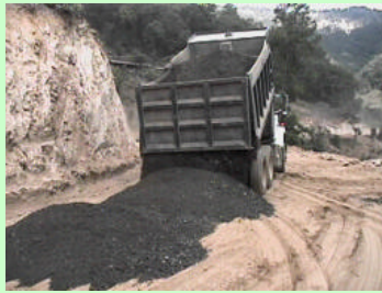
Adding 1 1/2" minus crushed volcanic rock
